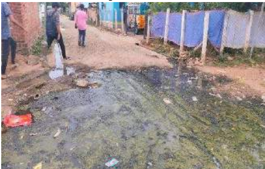
Sewage water on roads
